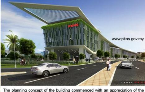
The low-energy approach involved orienting the building north-south; thus reducing exposure to direct sunlight. Breaking the long building into series of smaller blocks allowed more natural light in, therefore reducing dependence on artificial lighting.
